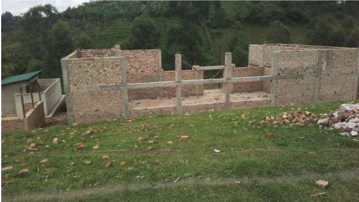
A Coffee huller under construction in Bitooma Sub-county, Bushenyi
