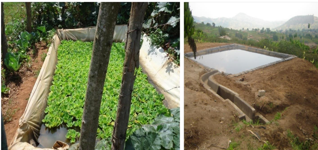
Figure 5-9 Underground tanks: Tarpaulin lined tanks (left); HDPE Dam lined tanks (right)
