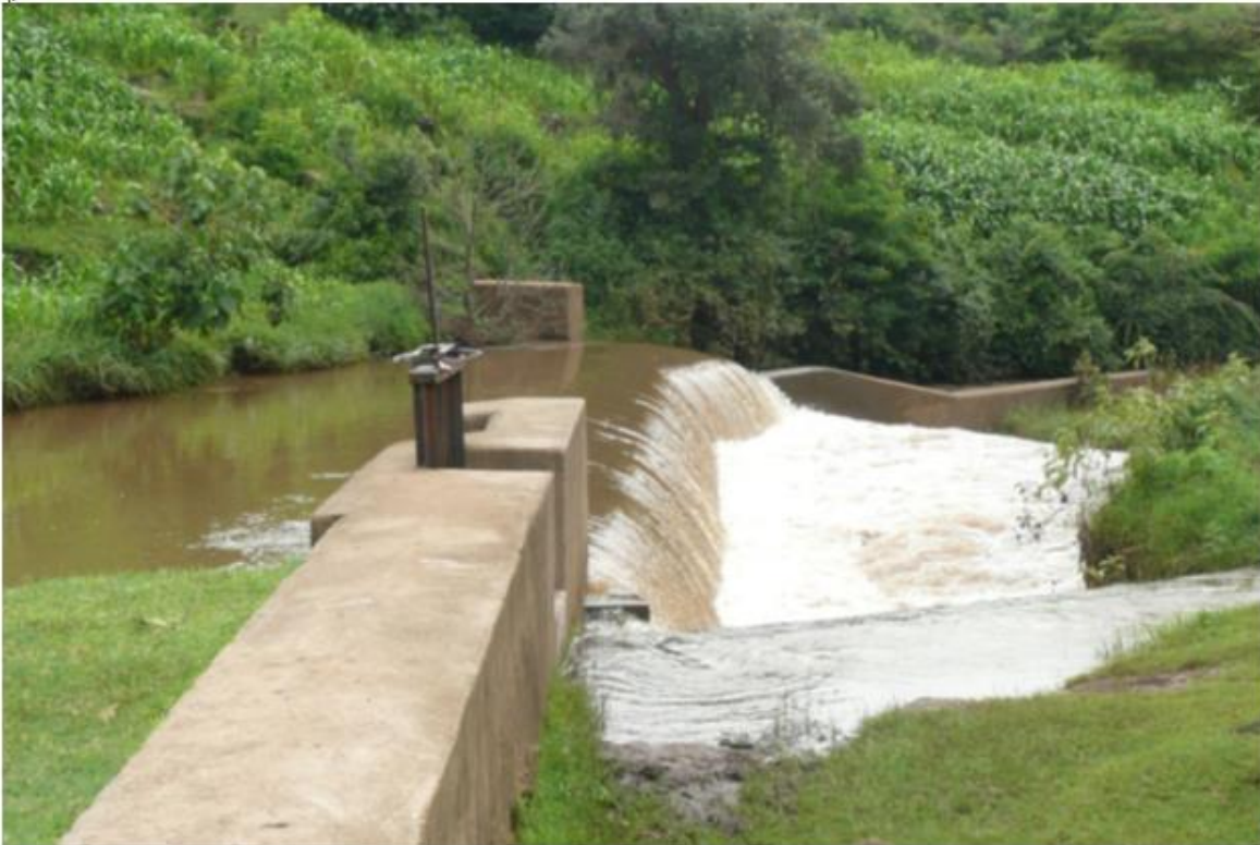
Figure 5-1: Typical river diversion works (concrete weir)
