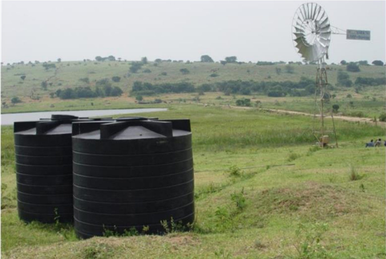
Figure 5-15 Wind mill for groundwater abstraction
