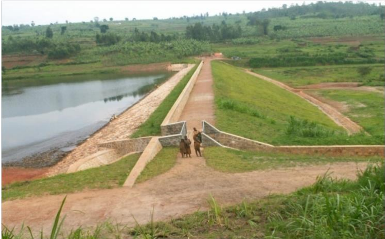
Figure 5-3 Small earth dam
