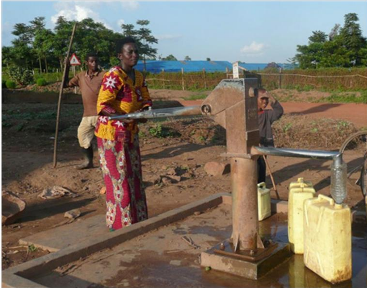
Figure 5-10 Suction hand pump (Source: Mati 2012)
